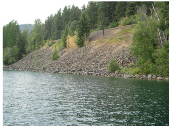
Figure 4. Sidecasting at Mackinaw Bay.
