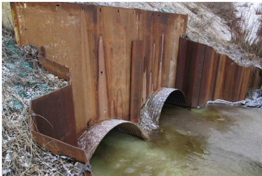
Figure 80. Haskill Creek Culverts on Monagan Road.
