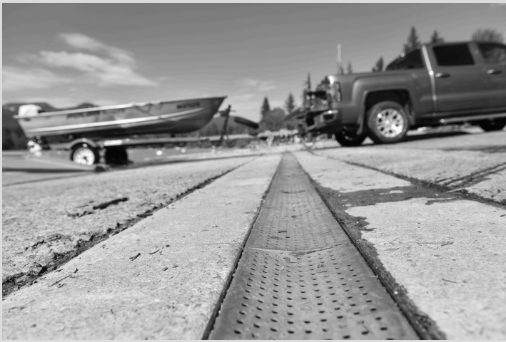
The interceptor trench installed in 2014 at the boat launch is designed to capture contaminants before they reach the swimming public at Whitefish City Beach.
