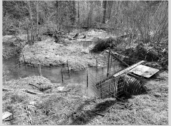
WLI partnered with Montana FWP, Montana DOT, and the National Wildlife Federation to install a beaver exclusion fence near Viking Creek to reduce flooding while supporting healthy wetland habitat.
