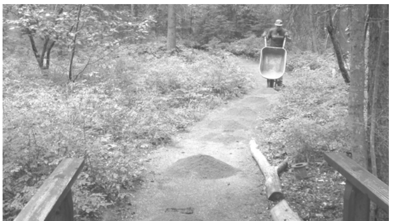
Thanks to a grant from the Montana Fish, Wildlife & Parks Recreation Trails Program, the trails and forest in Averill's Viking Creek Wetland Preserve are receiving a face lift. Last fall, crews from Forestoration repaired and resurfaced the trail with crushed stone. To improve safety, Forestoration sawyers cut standing hazard trees from the trail corridor. This spring crews will conduct management of noxious weeds.
