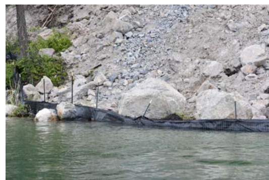
An ineffective silt fence in the lake was replaced with a WLI recommended turbidity curtain to limit fine sediment delivery to the lake.
