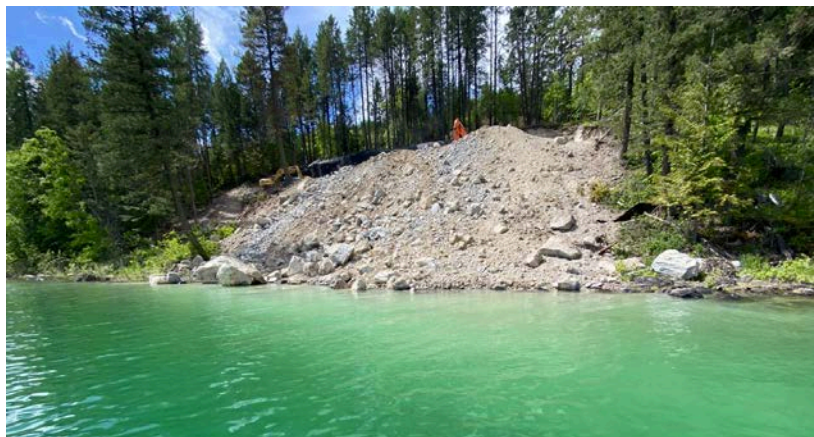
Blasted material covers a hillslope contributing unwanted fine sediment to Whitefish Lake.
