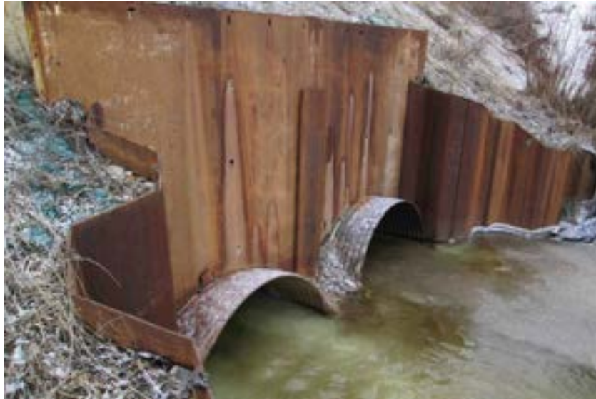
Figure 80. Haskill Creek Culverts on Monagan Road.
