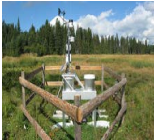
Figure 28. WLI Weather Station/Bulk Loading.
