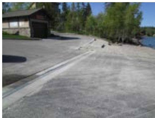
Figure 26. City Beach Boat Ramp Trench. Photo Courtesy WLI
