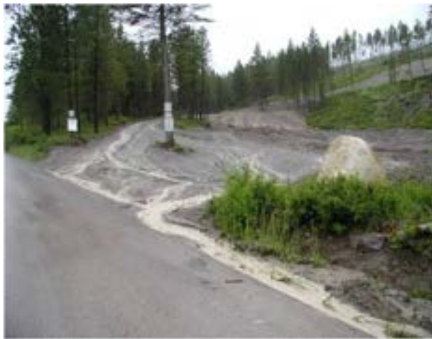
Figure 3. Erosion from Improper Development. Photo courtesy WLI
