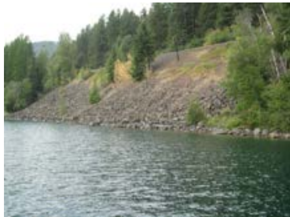
Figure 4. Sidecasting at Mackinaw Bay.
