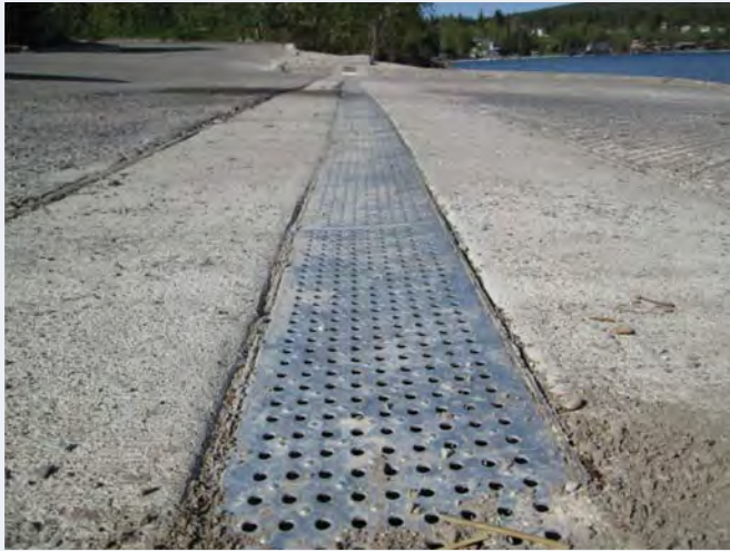
Interceptor Trench. Photo courtesy Whitefish Lake Institute
