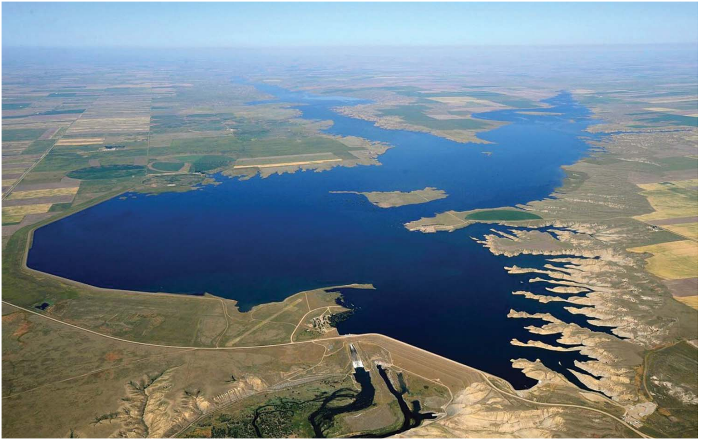
Tiber Reservoir and Dam. Photo courtesy www.larrymayer.com
