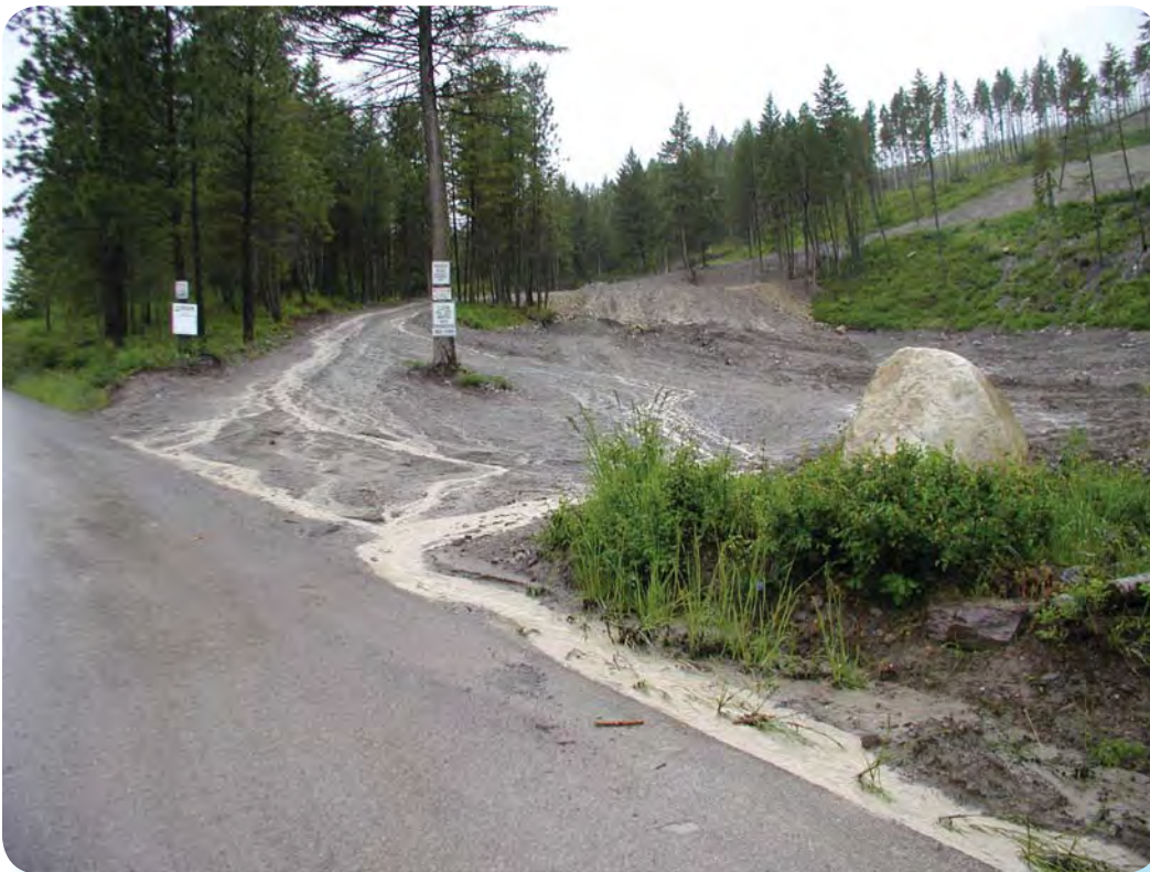
Poor road building practices. Photo courtesy Whitefish Lake Institute
