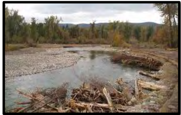
A reconstructed reach of the Jocko River illustrating channel shaping, large wood habitat structures, and vegetated soil lifts.
