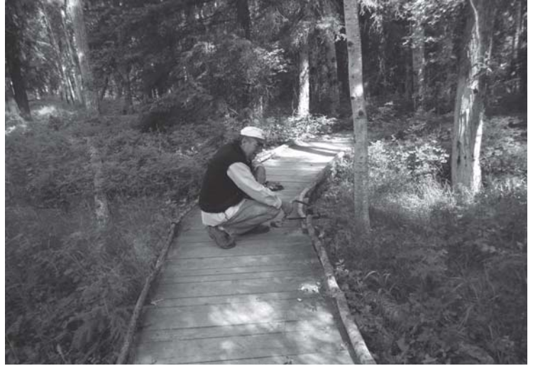
Wetland Work Day volunteer Walt Curtis replaces a toe kicker on a boardwalk segment of the Living Wetlands Interpretive Nature Trail .
